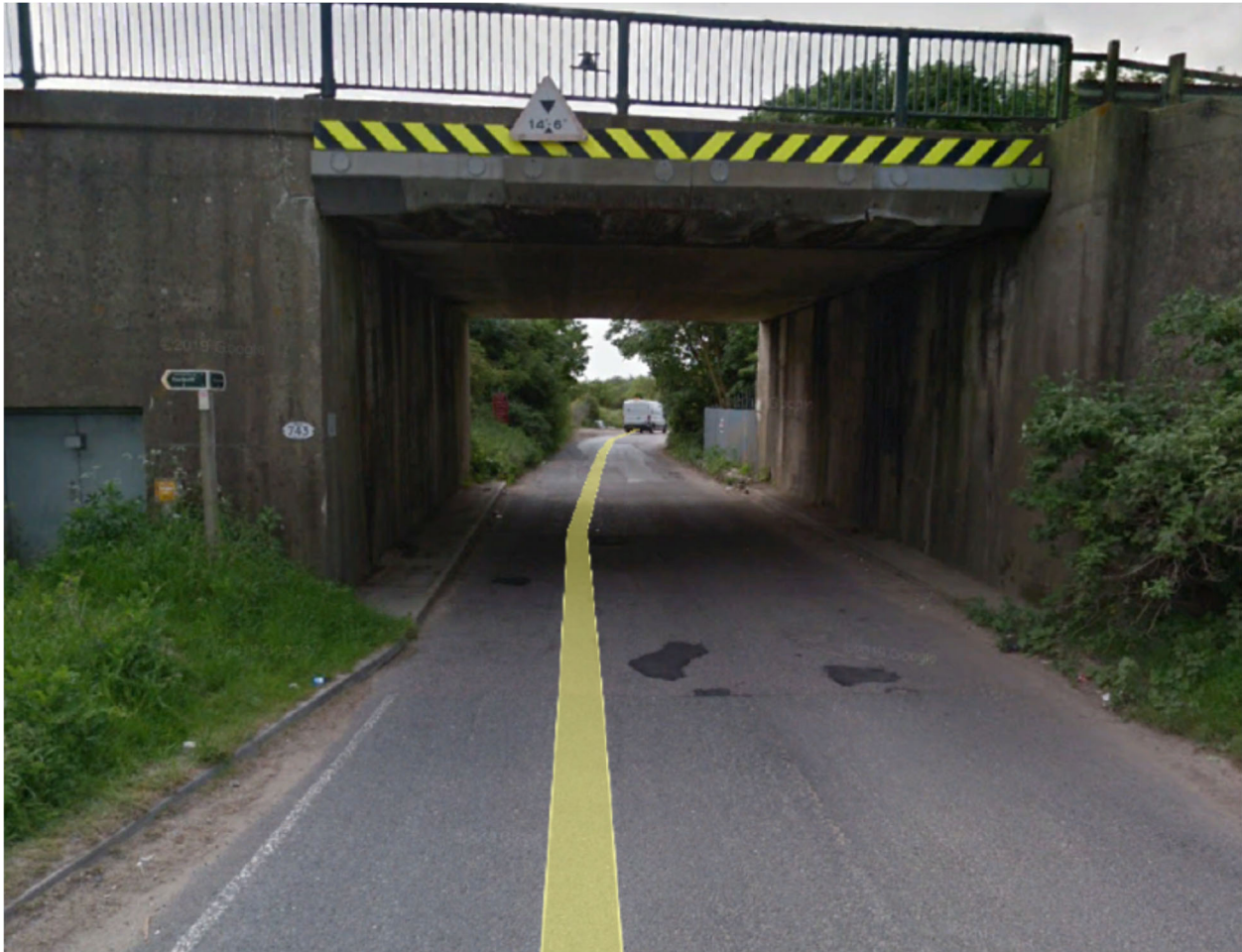
Figure 1: Railway Bridge over Western Access Road
